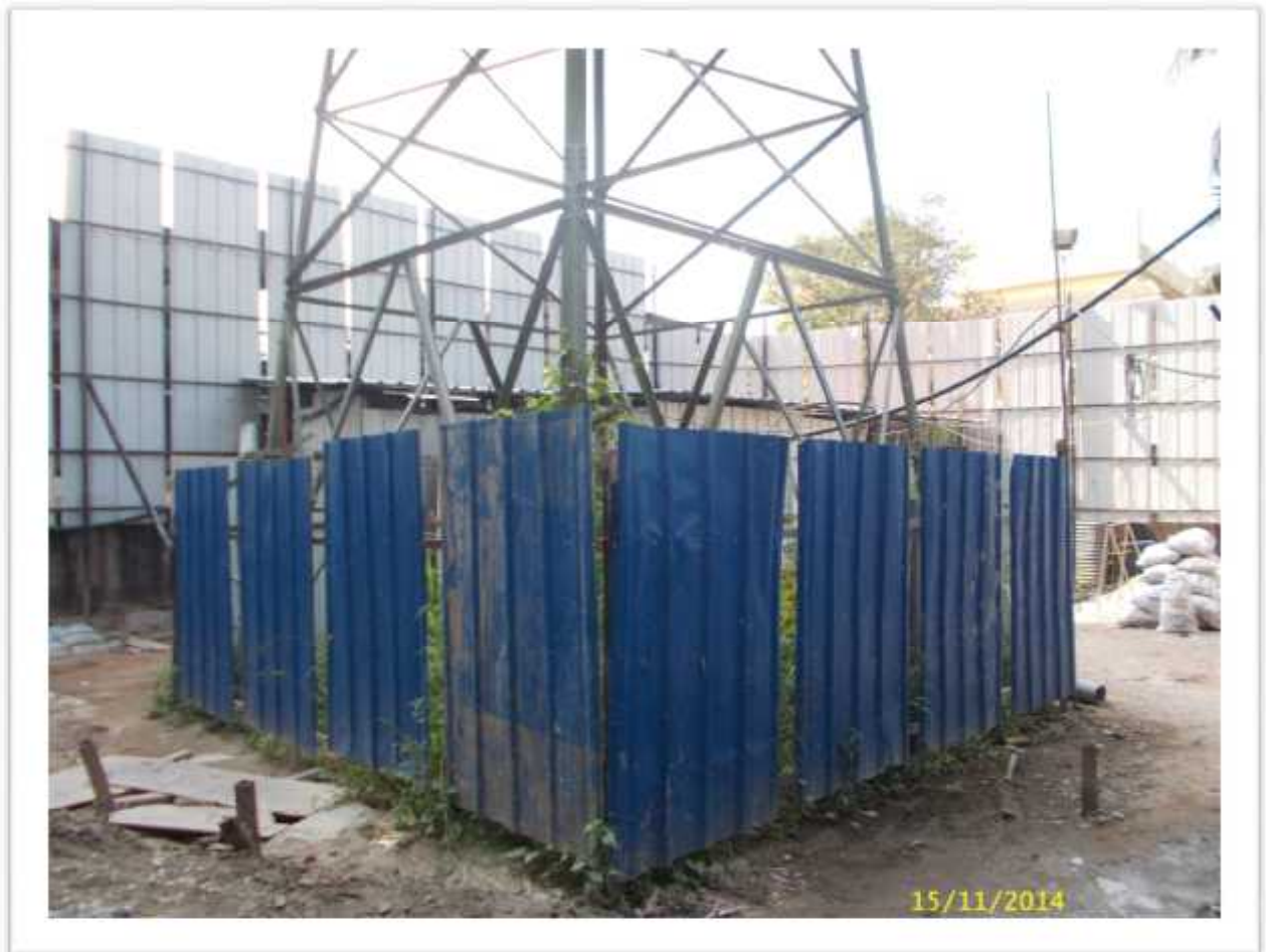
Photograph for the fencing provided around the tower line
